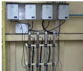
UV system for disinfection of chemicals 4x VAP SD 75 for 1m 3 /h Brazil
