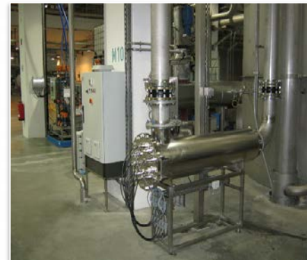
UV system for disinfection of process water UXP P 4400 (340 m 3 /h - 40°C) Germany
