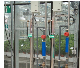
UV system for disinfection of process water in horticulture VAP SD 60 I for 200l/h Germany
