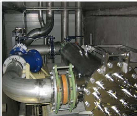
UV system for disinfection of process water UXP P 4400 (340 m 3 /h) Germany
