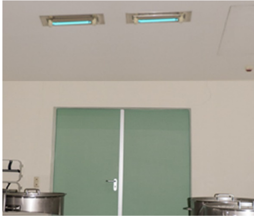
UV system for disinfection of air in storage rooms in the cosmetics industry Germany
