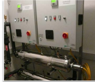
2 x UXPM OX 7000 E for the removal of cyanide in groundwater, Germany
