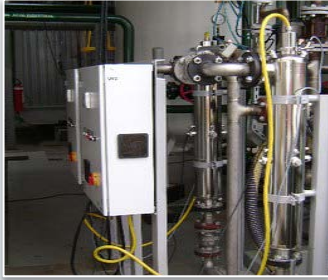
2 x UXPM OX 7000 E for AOP treatment in process water Brazil
