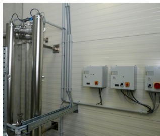
UV system for disinfection of process water 2x VAP-P 360 for 76m 3 /h Germany
