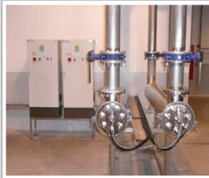
UV system for disinfection of process water 2 x UXP P 3200 (2 x 168 m 3 /h) Germany
