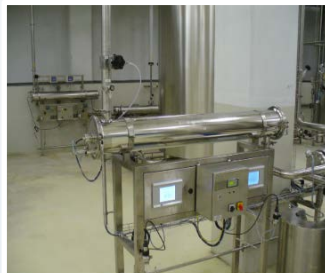
UV system in pharmaceutical design for residual ozone destruction
